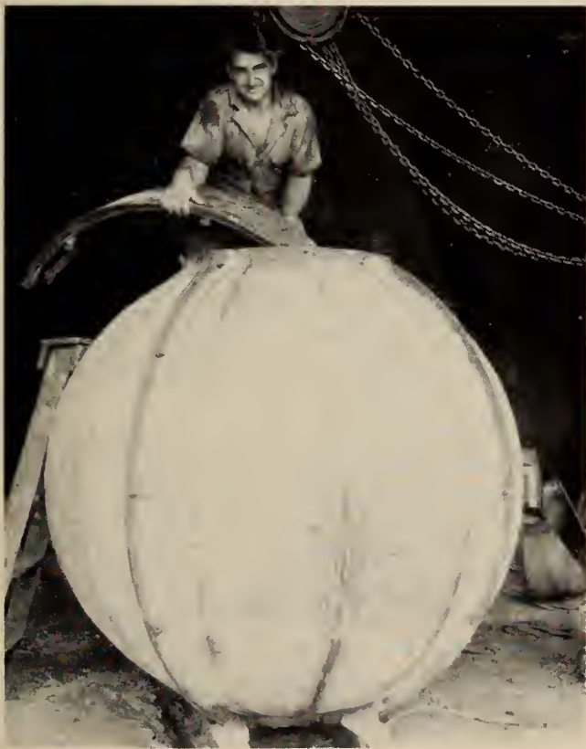
Segments of inside mold are removed through the manhole.
